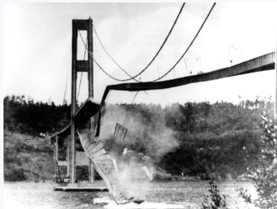
Figuur 50 – Instorting van de Tacoma bridge (bron: https://www.businessinsider.com/biggest-structural-failures-disasters-history-2019-11?r=US&IR=T ).
